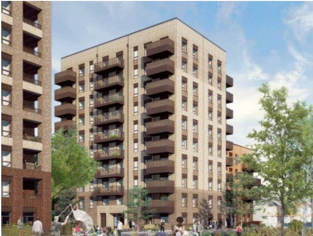
Image: view of Block A from the centre of the site
